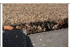
Base installation sub-standard, so resin surface will crack and ripple when vehicular weight on top think of icing on a sponge cake!
