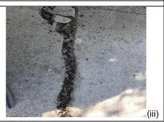
This Resin Bound Aggregate surface had been down 5 years: issues began almost at once – i.e. cracking, crumbling, wearing of surface showing tarmac base:
