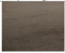
Trowelling / Floater marks, where the inexperienced floater has left marks in the finished Resin surface, usually as a result of
